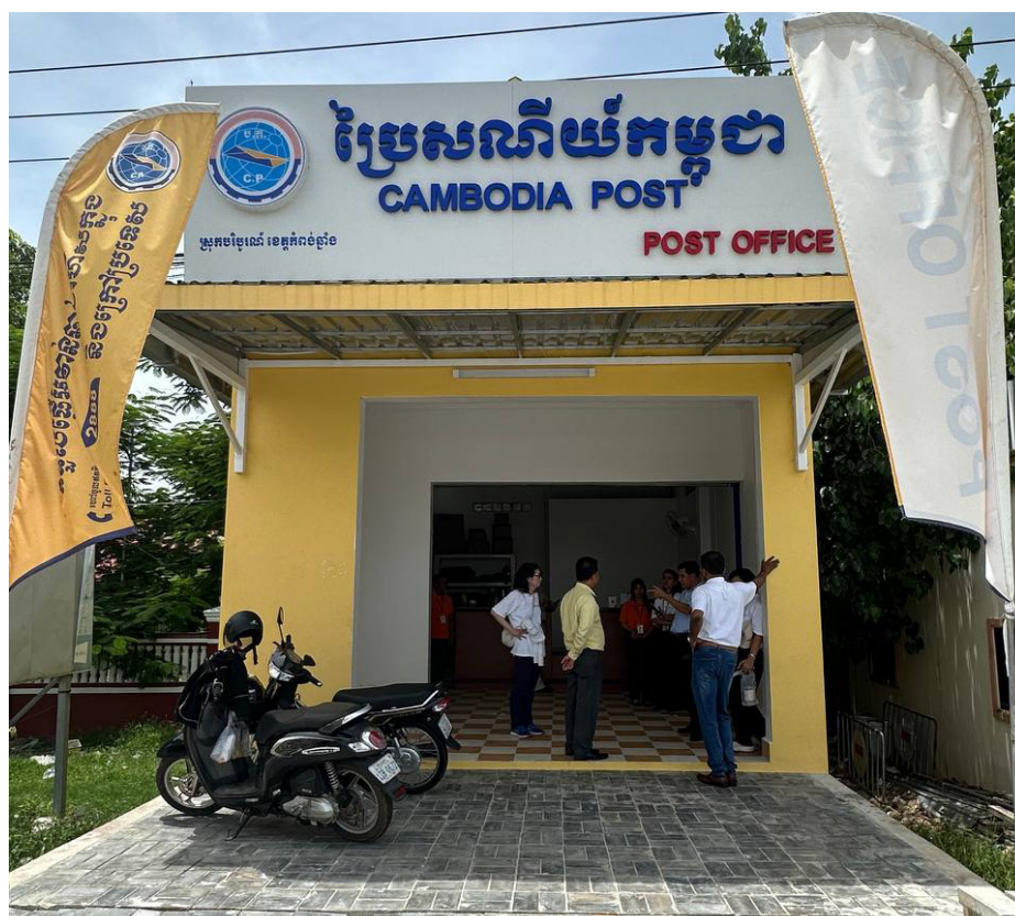
A newly constructed Cambodia Post office in a flood prone area.
