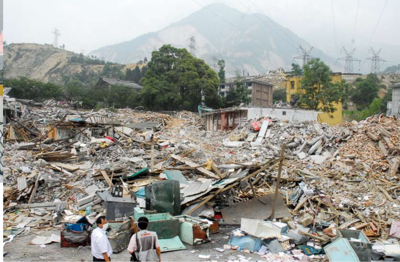
Ruins of a branch post office in Yinxiu county
